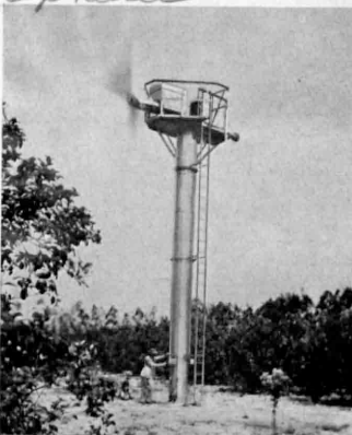
FOR FROST PROTECTION —Giant fans such as this one are replacing smudge pots to protect the fruit from frost in America's citrus groves.
