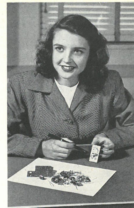
NEW-TYPE HEARING AID—The tiny "printed" circuit held by the young woman replaces the 173 items in the foreground which constitute the present hearing aids.
