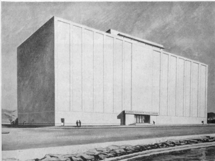
RADIOLOGICAL DEFENSE LABORATORY —The Navy's new laboratory for research on defense against atomic weapons, a six-story, windowless structure now being built in San Francisco, will look like this when completed.
