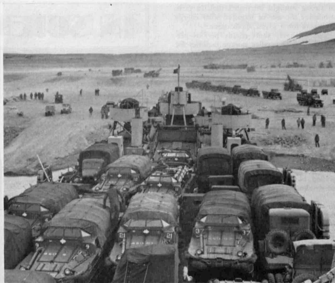
ARCTIC CIRCLE BASE —At Thule, Greenland, 900 miles from the North Pole, personnel unload vehicles to be used in construction of the new large air base there.
