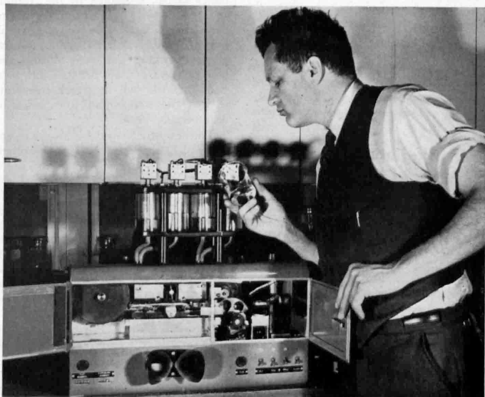
SPLIT SECOND PHOTO —This apparatus contains a camera which will take a picture in a millionth of a second and a developer that takes only 25 seconds. A projector throws a picture on the circular screen at the right end.
