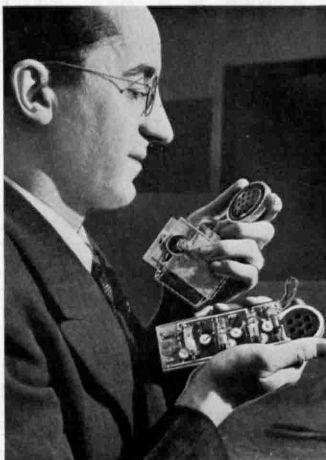
BROADCASTING AND LISTENING —Complete radio broadcasting station is held in the left hand of Dr. Cleo Brunetti of the National Bureau of Standards while a four-tube radio receiver is in his right.
