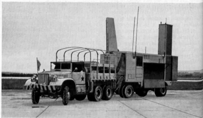
RADAR ON WHEELS —Mobile radar Ground Control Approach units such as this used by the Army Air Forces, are being installed in commercial airports.
