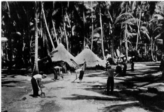
"MAIN" STREET—Seabees lay down steel mats which are later filled with coral rock to make a smooth surface for the main street at a Southwest Pacific Navy base. In the background are the Seabee tents hidden from sight of enemy planes by towering coconut palms.
