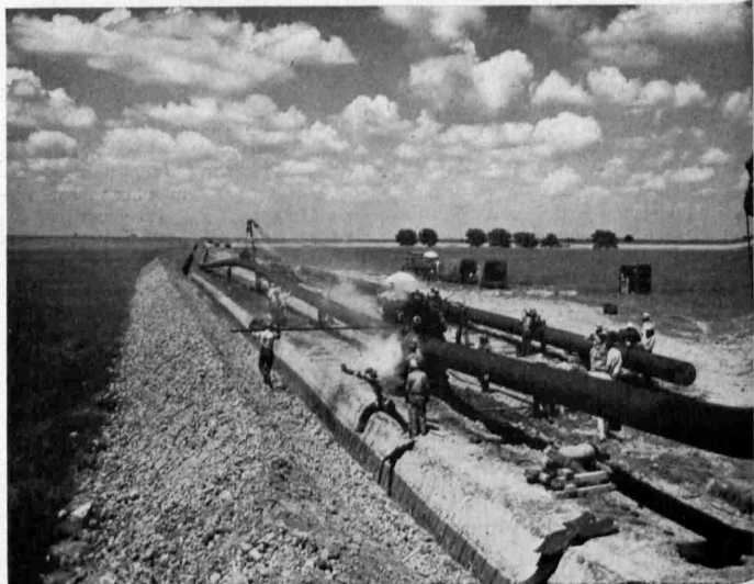
WILL CARRY GAS —Before it is dropped into the trench, a protective coating is put on the pipe of the Tennessee Gas and Transmission Co., destined to carry natural gas to the Appalachian industrial areas
