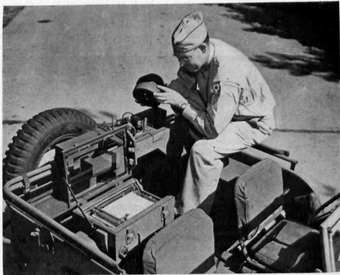
MECHANICAL MAP MAKER —The land Odograph automatically plots the course travelled by this jeep, providing valuable military reconnaissance information for field commanders. Captain Faustman of the Army's Engineer Board holds the cover of the electronic magnetic compass which determines the direction in which the jeep is travelling. In the foreground is the mechanical plotting unit which controls the movement of the pencil on the map table.
