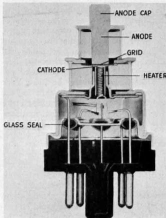
**"LIGHTHOUSE"** — This new disk-seal electronic tube, known to engineers as a megatron tube, developed by the General Electric Company's Electronic Laboratory, greatly advances the frequencies and power available to electronics and makes possible a new family of ultra-high frequency apparatus.
