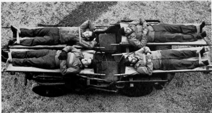
JEEP AMBULANCE —Another use has been found for that most versatile vehicle of the Army. How easily and efficiently it can be converted to carry four wounded men on litters is illustrated in this official U. S. Army Signal Corps photograph taken somewhere in England.
