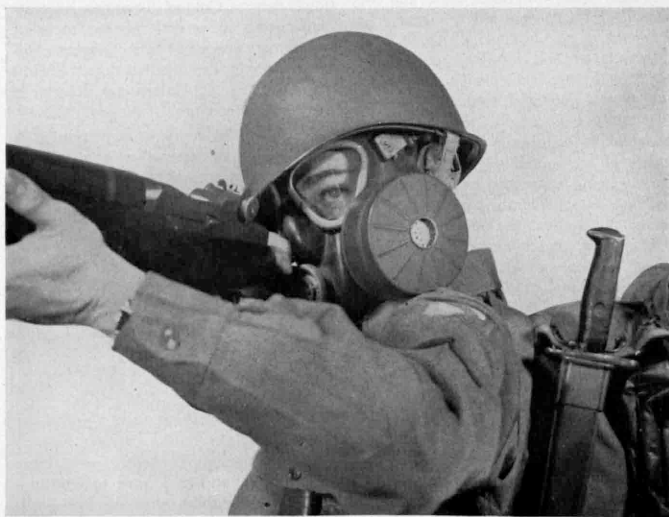
NEW TYPE —This lightweight "assault service" gas mask has recently been developed by the Chemical Warfare Service. Most striking difference in its appearance compared to the old type mask is the air-purifying canister protruding from the cheek of the mask.
