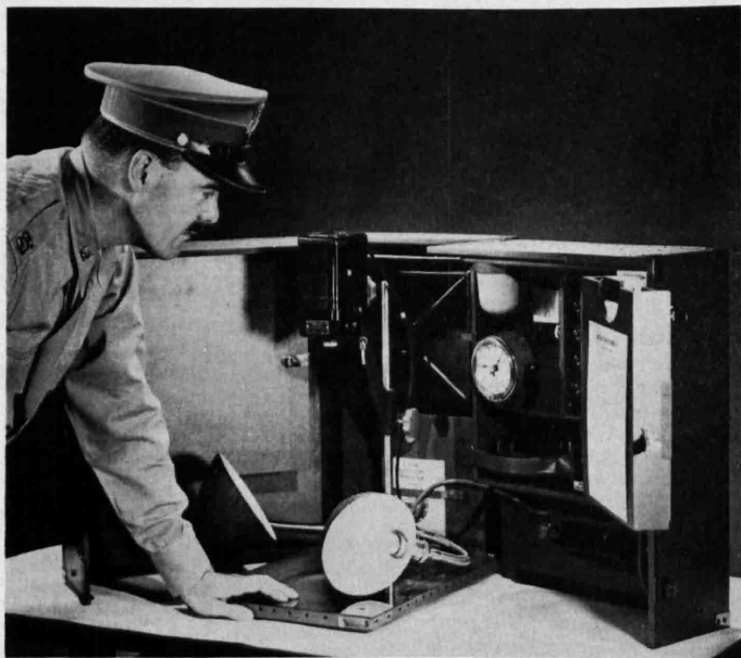
PORTABLE DARKROOM —Photographers for the armed forces can carry by hand this complete darkroom, housing all materials for taking pictures and processing them in a box less than two feet on a side. When necessary, daylight developing and printing can be carried out in a truck or tent. After the war a civilian model of the outfit will probably be available from Eastman Kodak.
