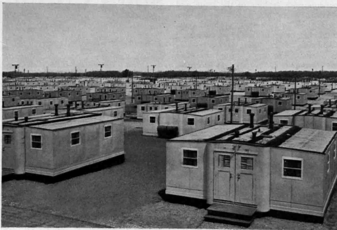
MOBILE HOUSING —These houses that can be folded up and moved elsewhere overnight are proving particularly useful in alleviating the housing shortage near new war plants.
