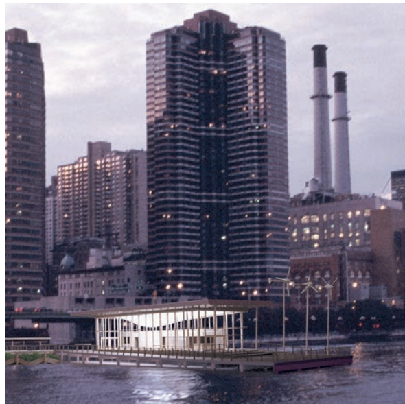
WIND POWERED — A photo composite of the New York skyline and an architectural model shows how LEDs could illuminate the ceiling on a landing for East River ferries serving Manhattan. Electricity generated by windmills at pier's end would be stored in batteries until needed to power the lighting. New York City agencies commissioned the plans.
