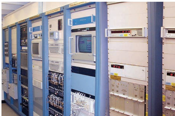
TICK-TOCK — The master clock system at the U.S. Naval Observatory in Washington, D.C., relies on a comparison of several dozen atomic clocks.
