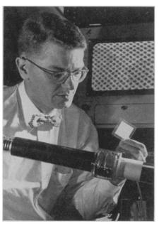
HONEYCOMB FOR COMPUTER— Dr. Harold R. Day, General Electric Research Laboratory scientist, holds a thin information storage mesh above the "reading and writing" tube in which it operates. The tiny honeycomb, with 250,000 holes per square inch, is electronically magnified on the television screen in the background.
