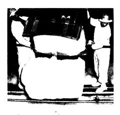
GLASS CLOUDS—A fibrous glass filter is being prepared to filter radioactive particles from the exhaust gases at the Hanford Atomic Products Operation. This bed of the fibers, seven feet deep and 56 feet long, is said to be more efficient and cheaper to operate than sand filters used in earlier designs.
